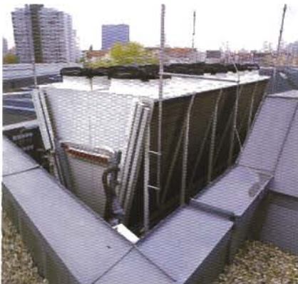
The V-shaped units are suitable when high capacity is demanded within restricted space.
